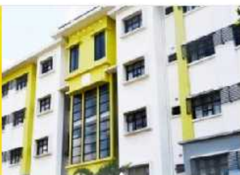
Dormitory Bumi Siliwangi fire/water
